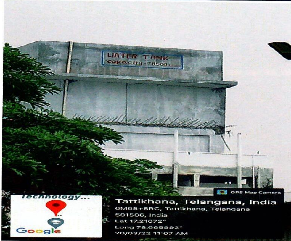
Overhead tank on Boys hostel.
