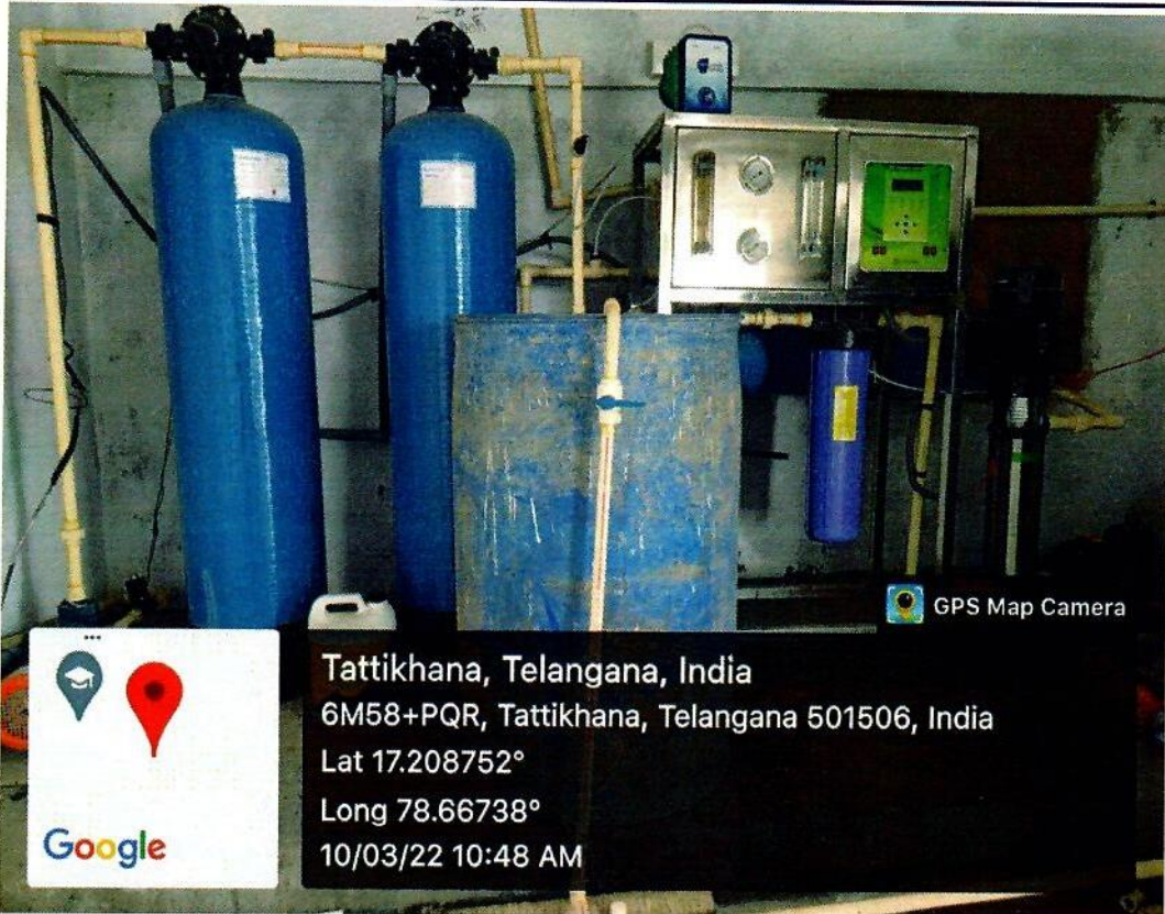
Ro plant girl's hostel
