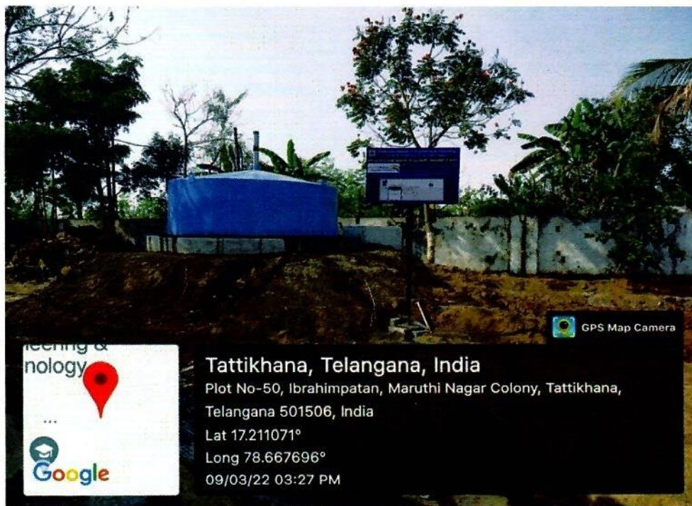
Biogas plant in college hostel.
